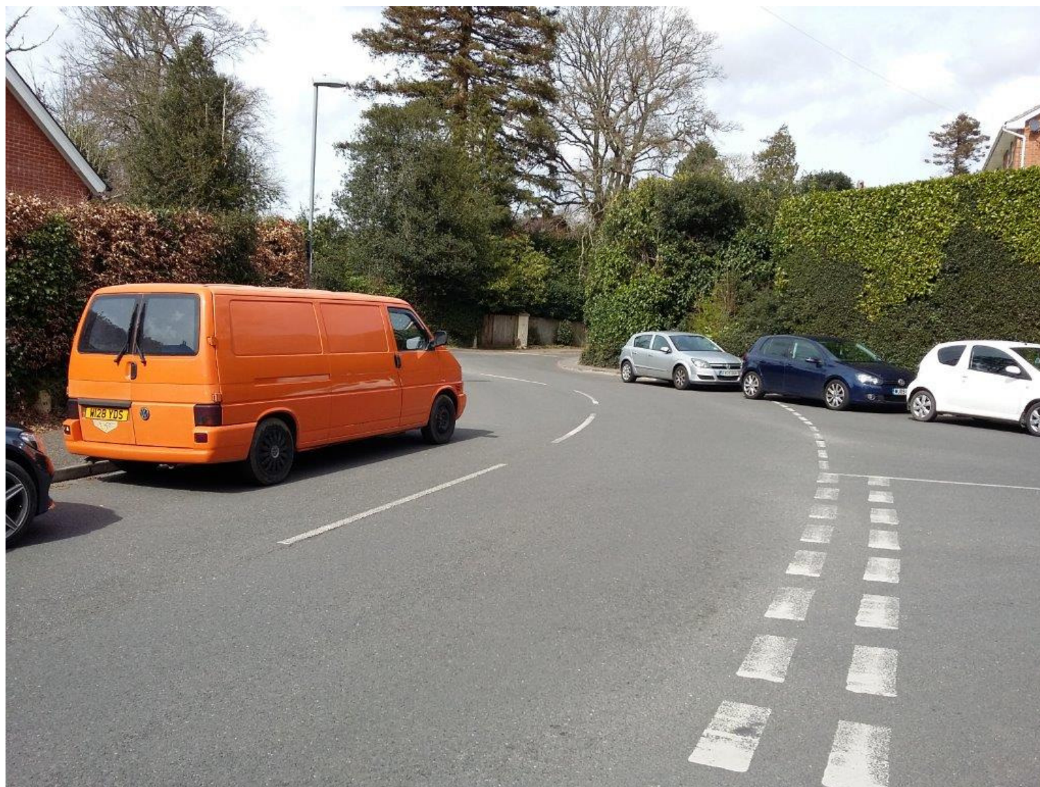
APPENDIX 2 another view looking northward from the junction of St Johns Hill with Cranfield Avenue towards the roundabout
